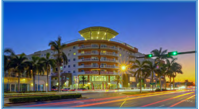
Dania Beach, FL - The Place at Dania Beach is a mixed-use project consisting of 144 luxury affordable housing units, ground-floor retail, rooftop recreation space, and an attached parking structure.
