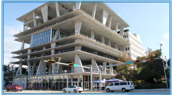
Miami Beach, FL - 1111 Lincoln Road Garage incorporates retail, office, parking, event spaces, and even public artwork
