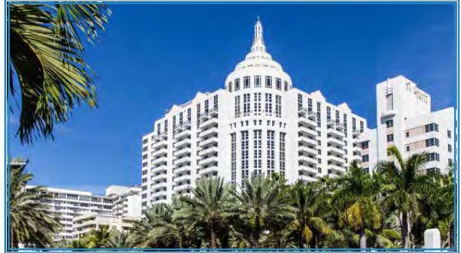
Miami Beach, FL - Built on land leased from the City, the Loews Miami Beach Hotel includes a publicly-accessible parking garage and a much-needed convention center.
