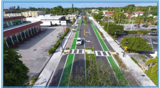
Fort Lauderdale, FL - Implemented Complete Streets design strategies, including a mid-block crossing, bike lanes, narrow travel lanes along NE 13 th St
