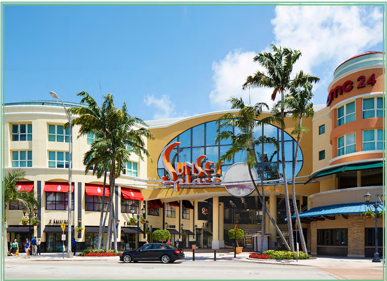
The Shops of Sunset Place prior to being redeveloped.
