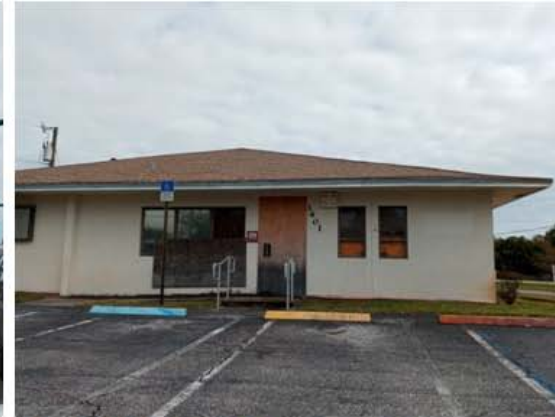
Abandoned Building at Davis Rd and 2 nd Ave
