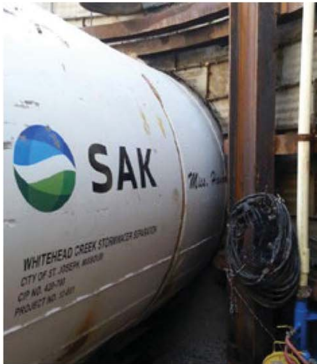
Large Diameter Tunneling
