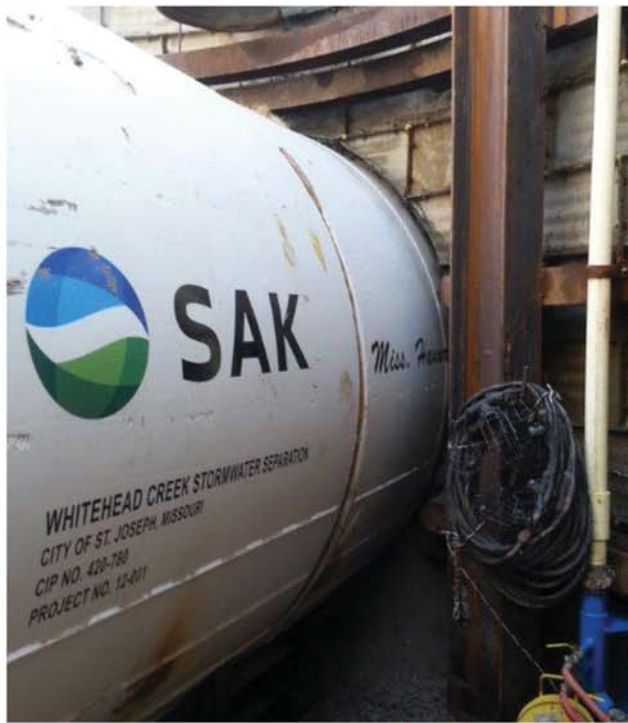
Large Diameter Tunneling
