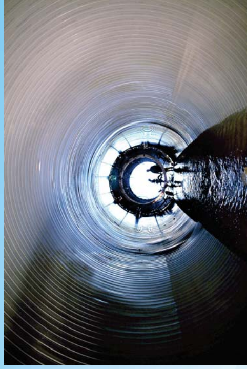
Spiral Wound (SPR) after rehabilitation
