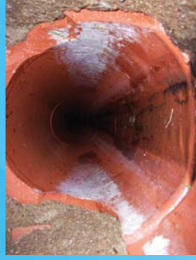
Before CIPP rehabilitation
