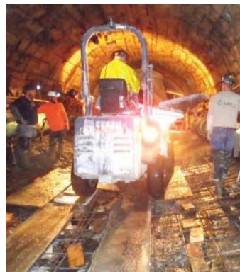
SAK Construction LLC, recently began work on rehabilitating a 5,575-lf segment of the Old Mill Creek Sewer in Downtown St. Louis.
