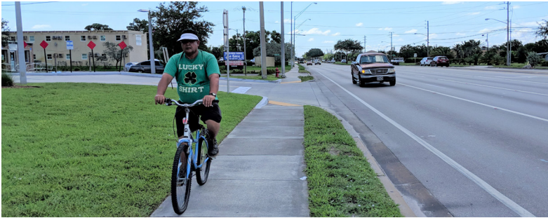
Typical sidewalk width along the north side of the street is 5’ with a 3’ planting strip, 2’ curb and gutter, and a 3’ shoulder at the edge of the roadway.
