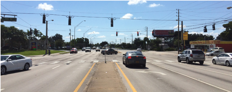
Lake Worth Road at Kirk Road. At signalized intersections, the wide landscaped median is reduced in size to accommodate left turn lanes.
