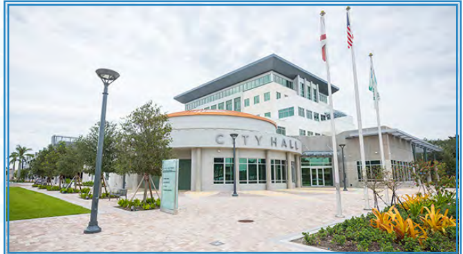
Coral Springs, FL - This City's newly completed municipal complex includes spaces for various City Departments, parking structures, and open spaces. The project also served as a catalyst for redevelopment.
