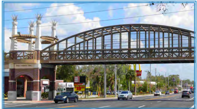
Apopka, FL - This pedestrian bridge allows pedestrians to safely cross over the busy West Orange Blossom Trail and serves as a gateway into the City's downtown.
