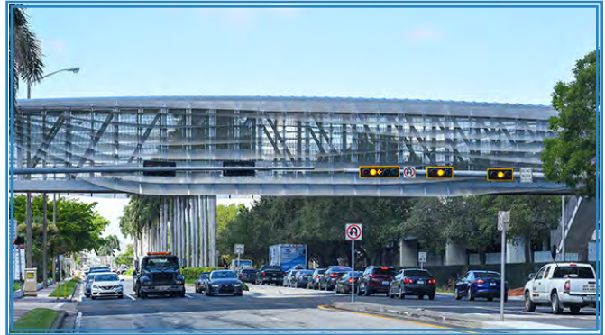
Miami, FL - Located a couple of miles northeast of the South Miami CRA, this pedestrian bridge allows pedestrians to safely cross U.S. 1.
