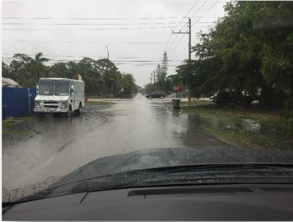
Looking north on Gulfstream Rd at intersection with 10 th Ave N
