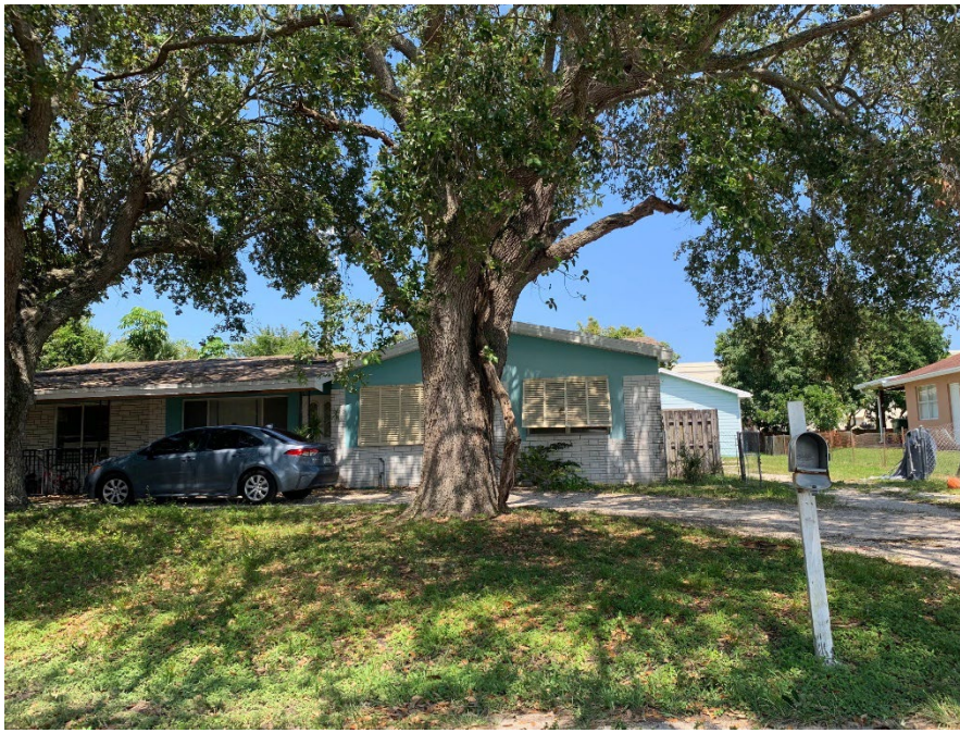
7 Existing structure on Lone Pine Way
