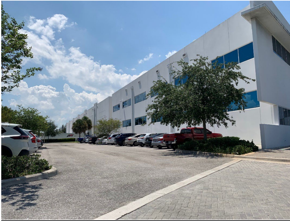
2_Northwest View of Existing Building
