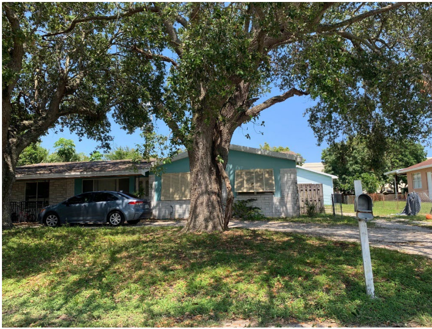
7 Existing structure on Lone Pine Way
