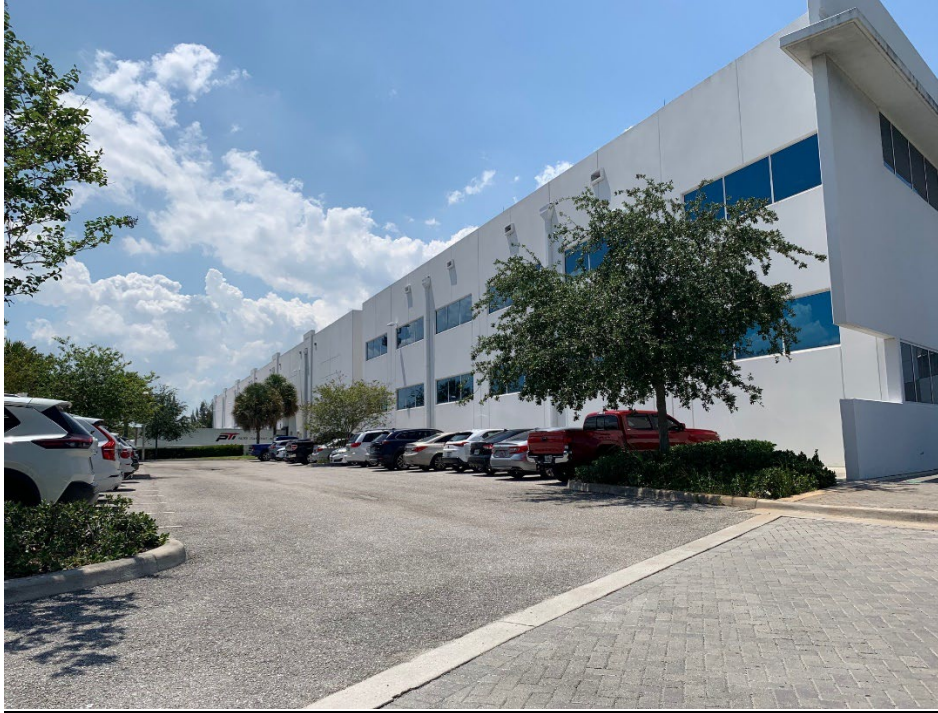
2_Northwest View of Existing Building
