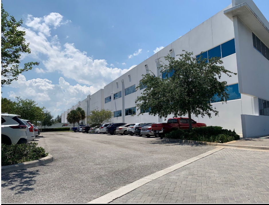
2_Northwest View of Existing Building
