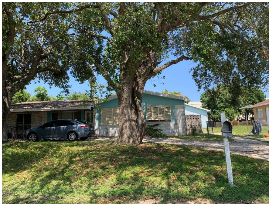
7 Existing structure on Lone Pine Way
