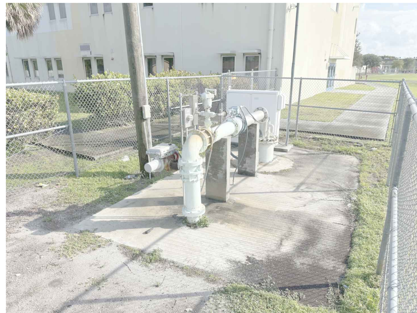
EXISTING WELL No. 14 SITE PHOTO
