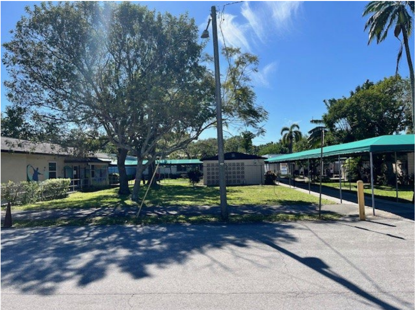
Figure 1 - Looking south at future parking lot location
