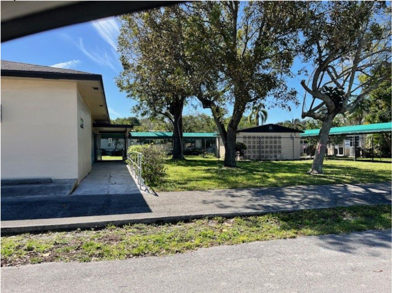
Figure 2 - Looking south at affected area
