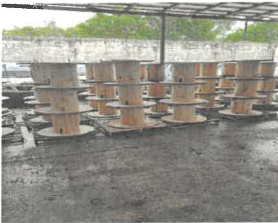
Example of outdoor storage Material
