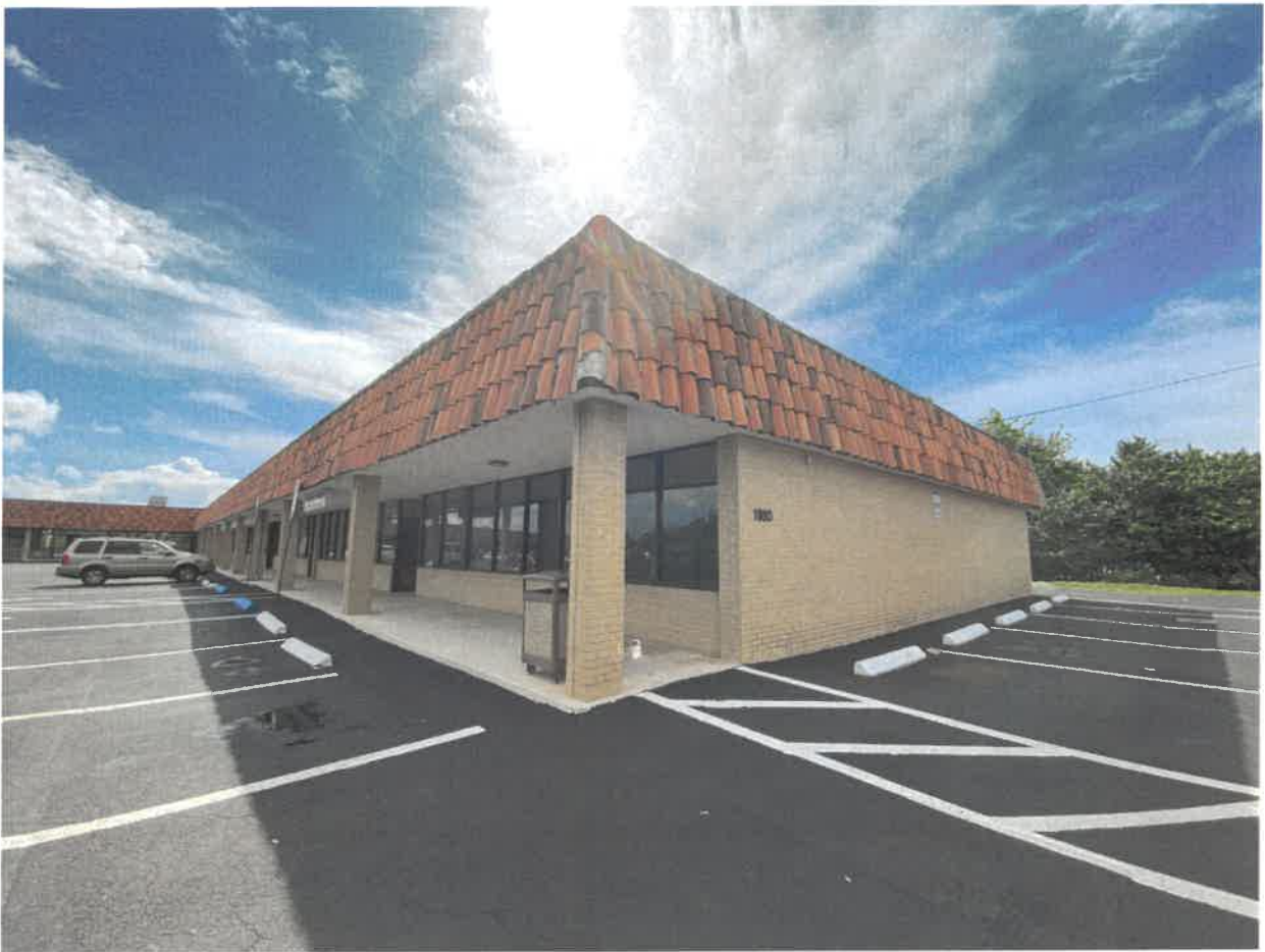
Sec. 10-9 Ext. Structure 9/24/2024 10:50:09 AM Fix Broken Roof Tiles
