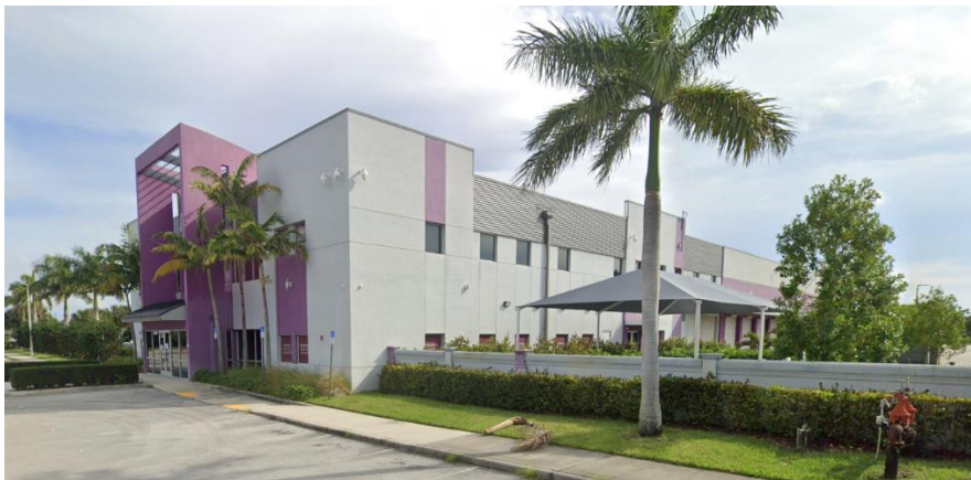
Main Building- South and West Elevation
