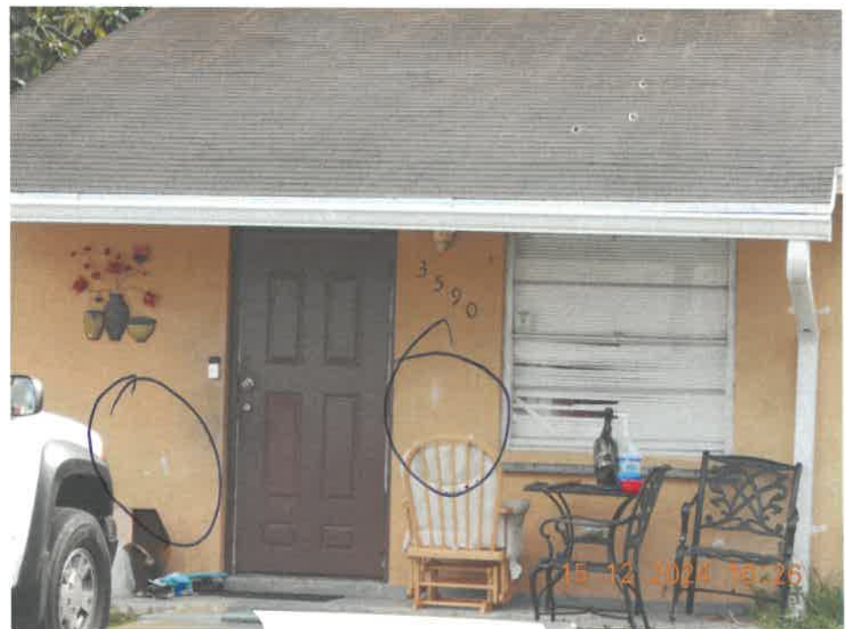
- Touch up small sections with paint.
