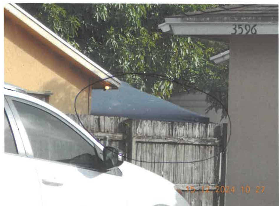
- Remove prohibited canopy.
