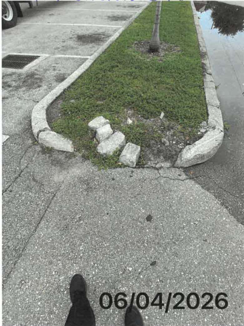
Repair Concrete Curb
